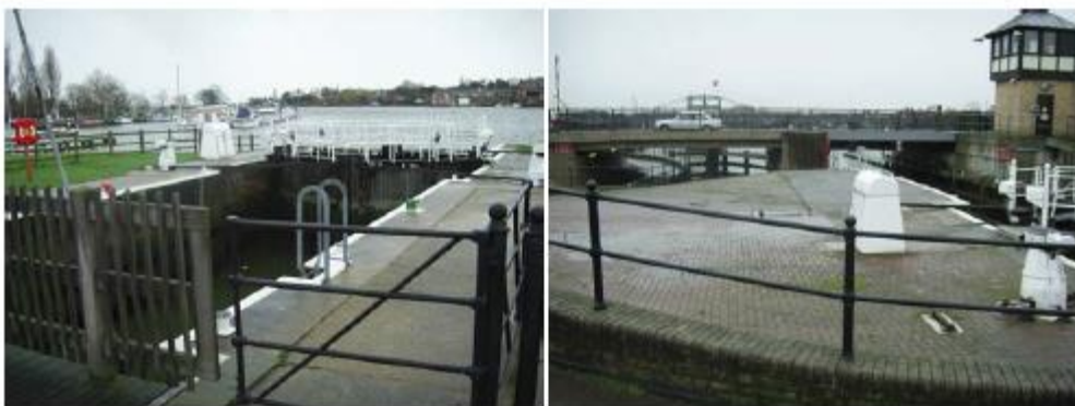
Plate 5-3 - Mutford Bridge lock gates acting as informal flood defences (extract from SFRA)
